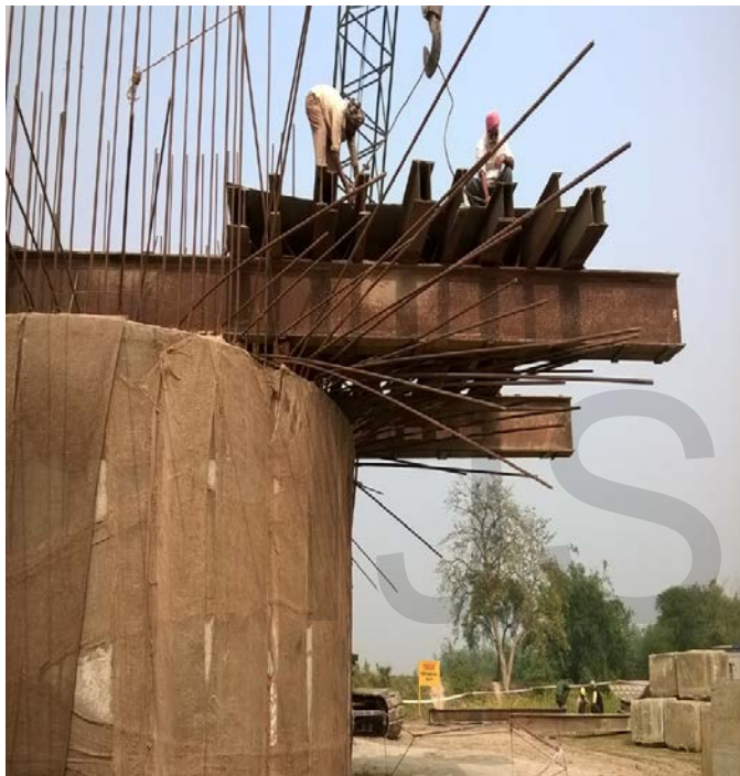
Figure 16- Fixing of Steel Girder for load placement
