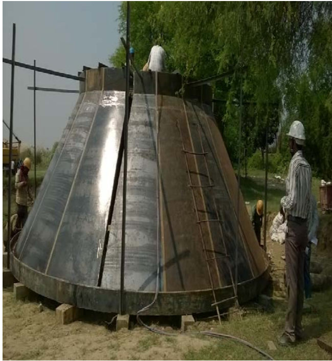
Figure 3- Inner Shuttering work for Well Curb
