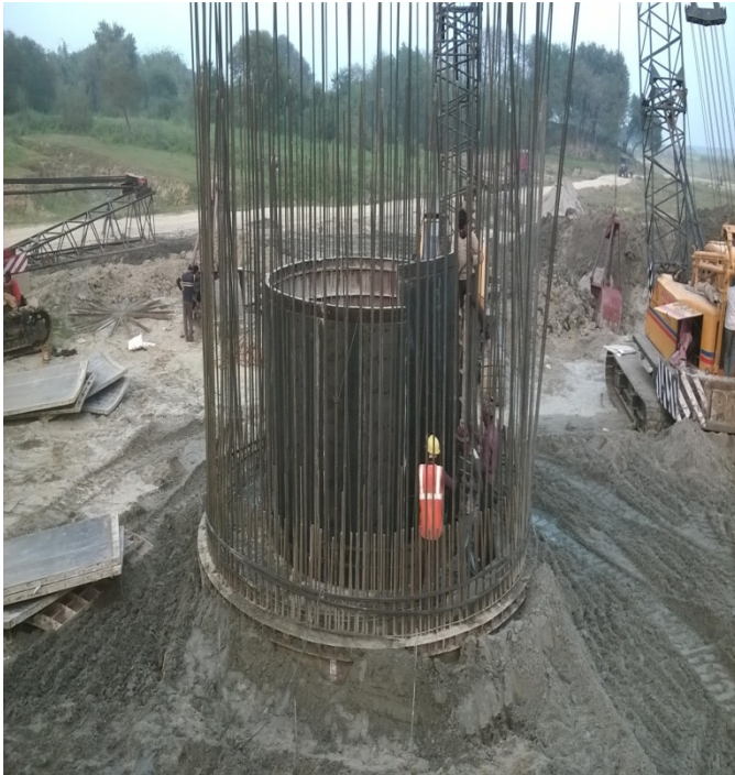
Figure 5- Shuttering work for Well Steining
