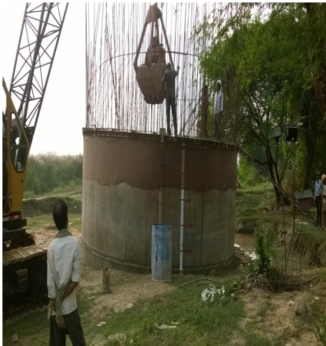
Figure 6- Sinking of Well Steining by Grabbing method
