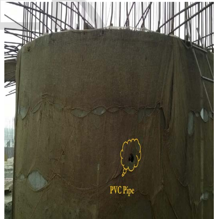
Figure 12- Provision of PVC Pipe (After casting of Steining)
