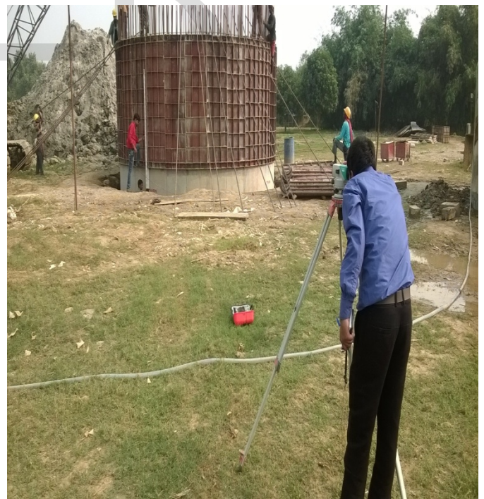
Figure 10- Tilt measurement by Auto Level
