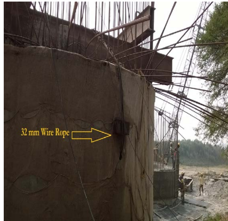
Figure 17- Anchoring of Steel Girders with Steining by Wire rope
