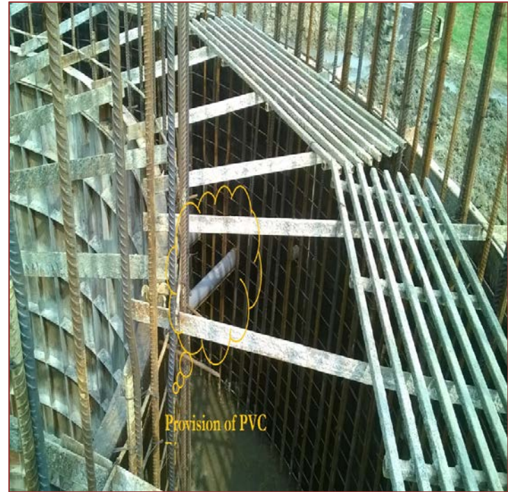
Figure 11- Provision of PVC Pipe (Before Casting of Steining)
