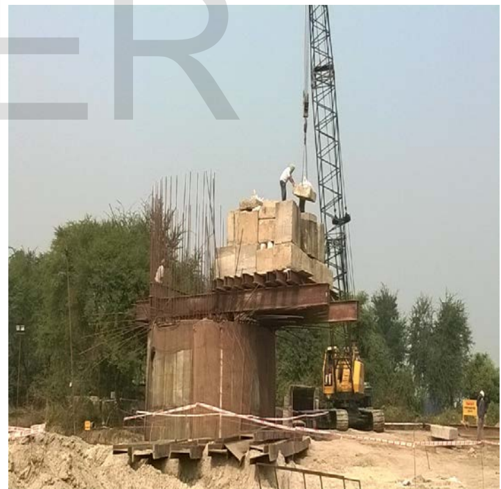
Figure 18- Kentledge Load Placement on Steel Girders
