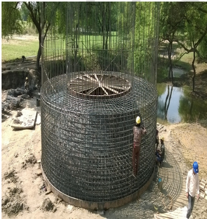
Figure 4- Reinforcement arrangement for Well Curb
