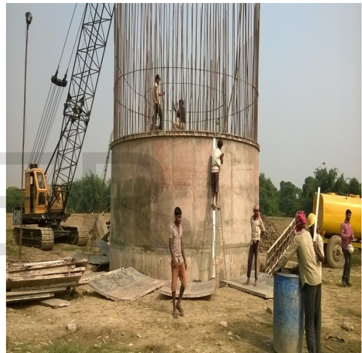
Figure 8- Gauge marking on Well Steining
