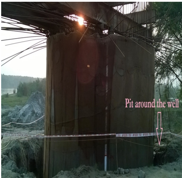
Figure 13- Pit around the well
